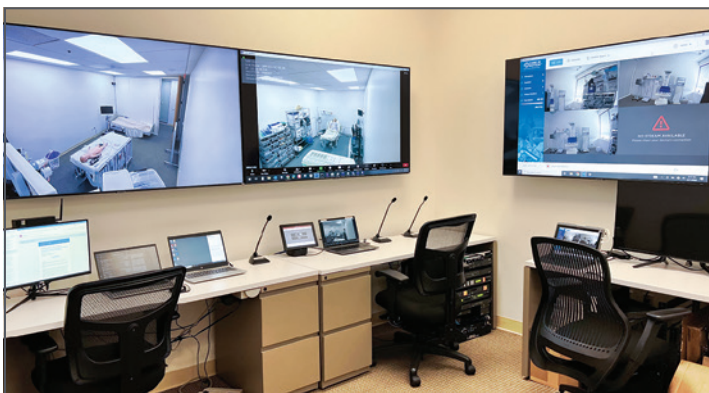
Simulation control room
